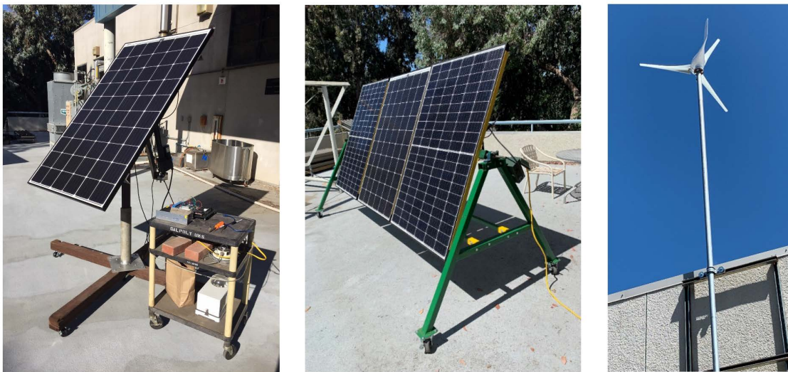
Figure 2: The micro-grid has three power sources. On the left, the dual-axis tracking solar panel. In the center, the adjustable fixed mount solar panel system that can accommodate up to three panels. On the right, the 400W wind turbine installed on the top of Building 13.
